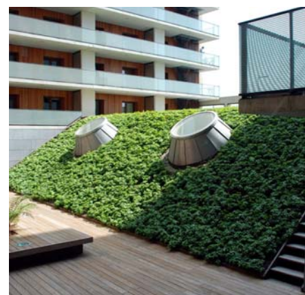
The maintenance of the lawn turned out to be costly. Therefore it was exchanged by a low maintenance ground cover planting.
