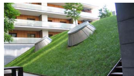
The pitched roof shortly after installation of the turf. Skylights allow for natural daylight inside the building.
