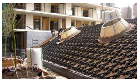
Two layers of Georaster® filled with substrate ensure proper supply of water and nutrients for the lawn.
