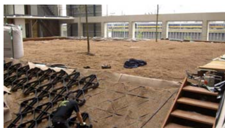
The proposed turf was intended to invisibly connect the pitched roof area to the flat roof area.
