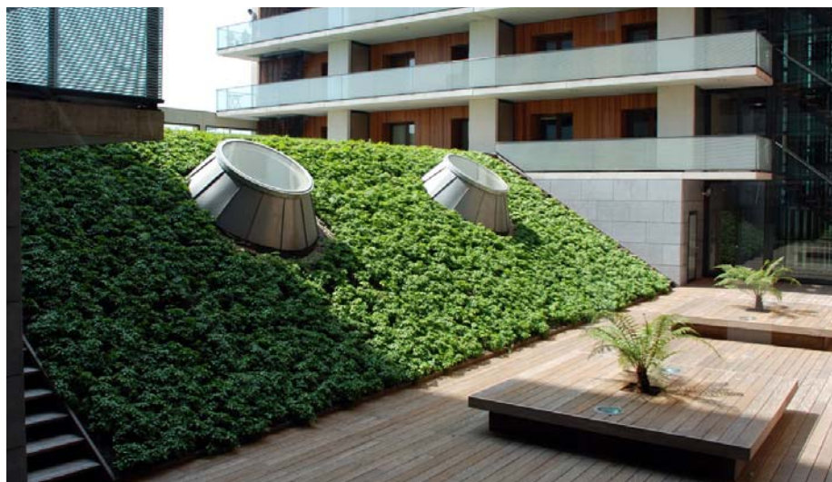
The inner courtyard of the "Australiëgebouw" with Pitched and Flat Green Roof.
