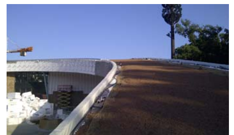
The system substrate suitable for lawn was applied in layer thickness of approx. 100 mm.
