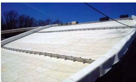
Shear retainers of the type Shear-Fix LF 300 and Eaves Profiles TRP 140 were installed in the steep roof areas in order to derive shear forces into the roof construction.
