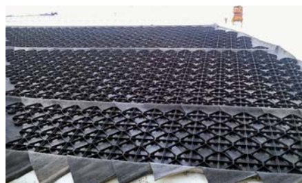
The synthetic Georaster ® elements, just before being filled with system substrate.
