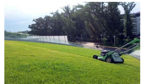
The green roof with its walkable lawn requires intensive maintenance including irrigation during dry periods.
