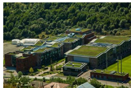
In 2015 upon completion of the school buildings the planners have received the International Green Roof Leadership Award for green roofs and walls.
