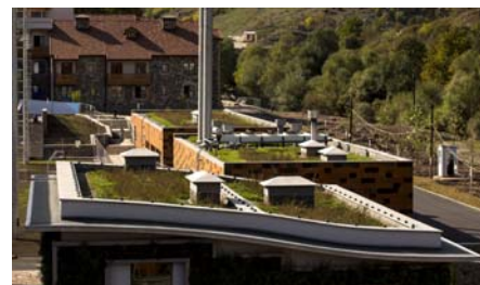
The plants on the roof surfaces are supposed to grow as naturally as possible.
