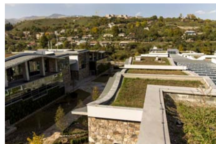
In order to preserve and increase biodiversity the roofs are mowed only twice a year.
