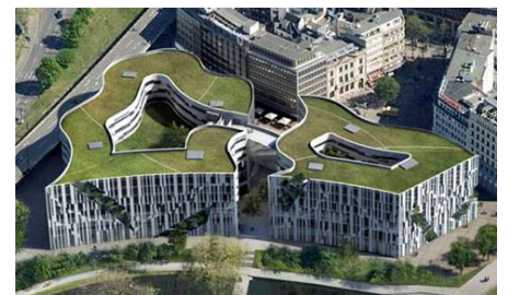
On the approximately 4.000 m 2 large roof surface the Floraset® FS 50 drainage element was installed. These elements are particularly suitable for large roof areas with little inclination and long drainage distances.
