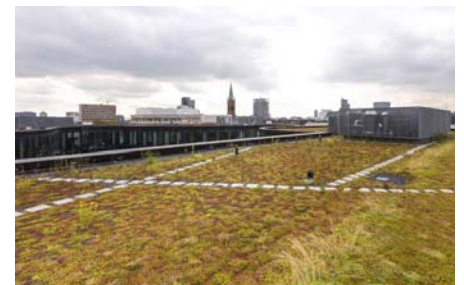
Pre-cultivated vegetation mats were applied along the edges whereas the centre of the roof surface was planted with Sedum sprouts.
