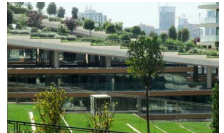
More than 200 different plant species, including 68 species of trees were planted on top and around the Zorlu Center.
