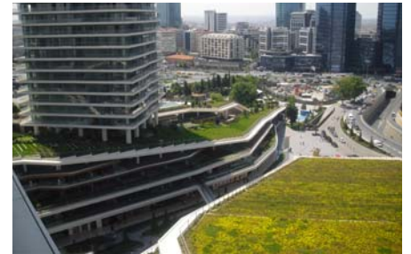
The intensive green areas with their shrubs and trees as well as the paved zones of the courtyard were all realized based on the Floradrain® FD 40-E drainage element, whereas the extensive green roof of the theatre is based on Floradrain® FD 25-E.
