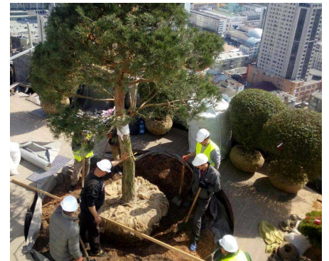
The latest Green Roof Technology enabled tall trees, such as Canadian Shadbushes, pine and maple (3.5–7 m), to be planted. A specially designed technological device which anchors the root ball of the central pine was used.
