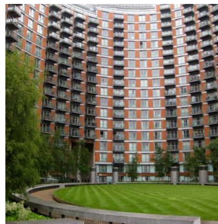
The inner courtyard with park benches above the underground garage.
