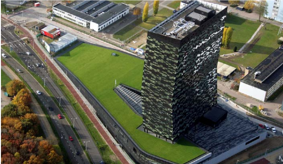
Aerial view of the FiftyTwoDegrees Business Innovation Centre in Nijmegen.
