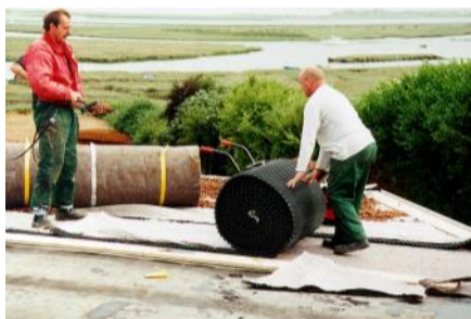
The Floradrain® FD 25-RV drainage element is provided in rolls and has an attached filter sheet SF.
