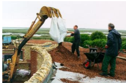
A blend of sedum carpet aggregate was applied as a growing medium for the vegetation mats.
