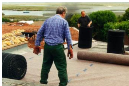
The protection mat SSM 45 was laid out as a base layer protecting the root resistant waterproofing.
