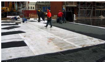
On top of the root-resistant roof construction of the parking garage the system build-up "Driveway" based on the drainage element Stabilodrain® SD 30 has been applied. This drainage element is quick and easy to be installed.
