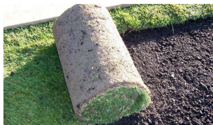
Pre-cultivated turf was laid on top of the substrate for quick covering.
