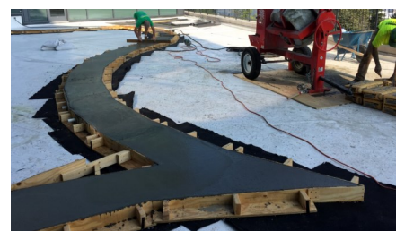
Floradrain® FD 40-E was used as a permanent formwork for the curb and seatwalls.
