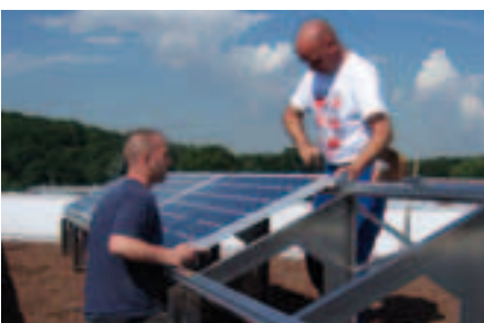
5. The solar panels are installed.
