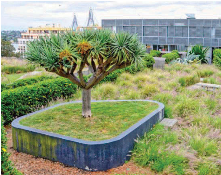
Intensive green roof, Sydney Photo: Matt Dillon
