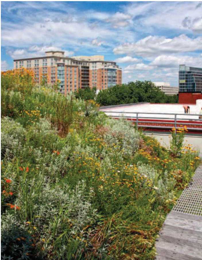
Extensive green roof, Washington, DC, USA.
