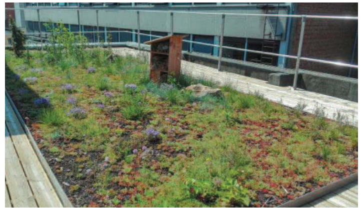
Blue green roof, Antwerp Photo: Vegetal ID
