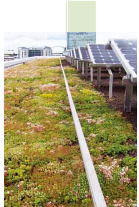
The classic area where a Fallnet rail system is used: peripheral areas, where work is required repeatedly. Once you've clicked into the runner, the work can be carried out in absolute safety.
