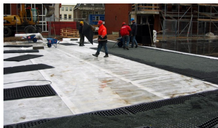
On top of the root-resistant roof construction of the parking garage the system build-up "Driveway" based on the drainage element Stabilodrain® SD 30 has been applied. This drainage element is quick and easy to be installed.
