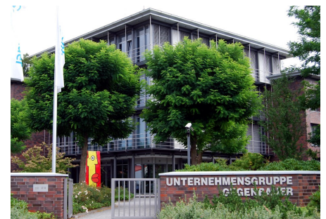
Unexpected sports activities take place on the 15 m high roof of this administrative headquarters of a company in Brandenburg.
