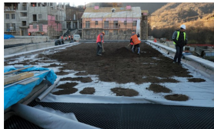
The substrate which was mixed on-site previously was applied all over the system filter.
