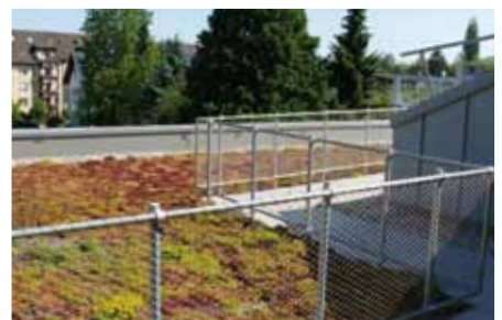
Individual balustrade solutions can also be mounted on the Guardrail Base. The connecting element in this case is the fixing flange. Otherwise, there are no limits to your creativity.
