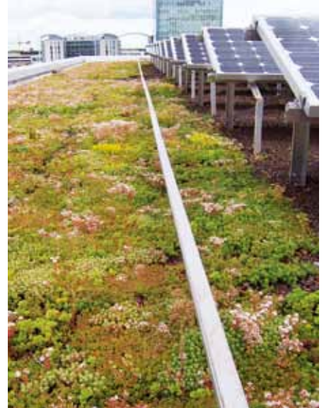
The classic area where a Fallnet rail system is used: peripheral areas, where work is required repeatedly. Once you've clicked into the runner, the work can be carried out in absolute safety.
