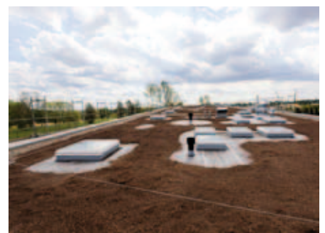
Installed system substrate "Rockery Type Plants".
