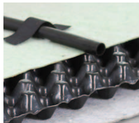
Velcro strips are used to attach the driplines to the Aquafleece.
