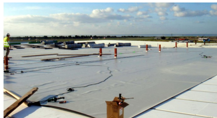
Preliminary work on the roof area to be vegetated.
