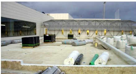
Protection mat, drainage elements and filter sheet are ready for installation.
