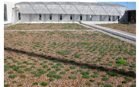
The roof area a few months after the plug plants have been planted.
