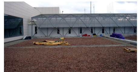
The roof area just after the application of substrate with BigBags.
