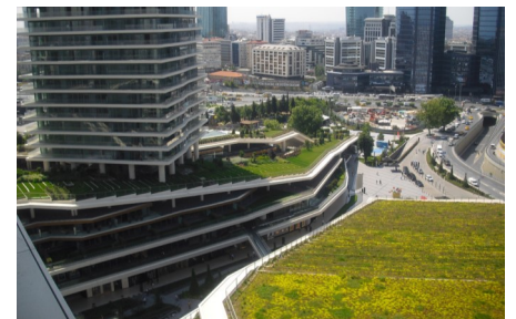
The intensive green areas with their shrubs and trees as well as the paved zones of the courtyard were all realized based on the Floradrain® FD 40-E drainage element, whereas the extensive green roof of the theatre is based on Floradrain® FD 25-E.
