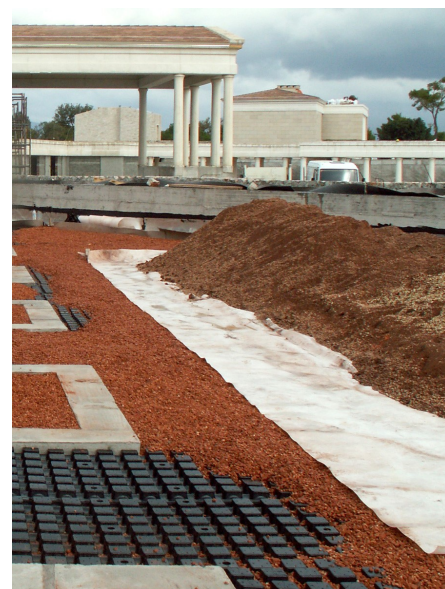
Floradrain® FD 60 elements were applied and infilled with Zincolit® Plus on this entire roof surface, also in the plant troughs which were meant for olive trees.
