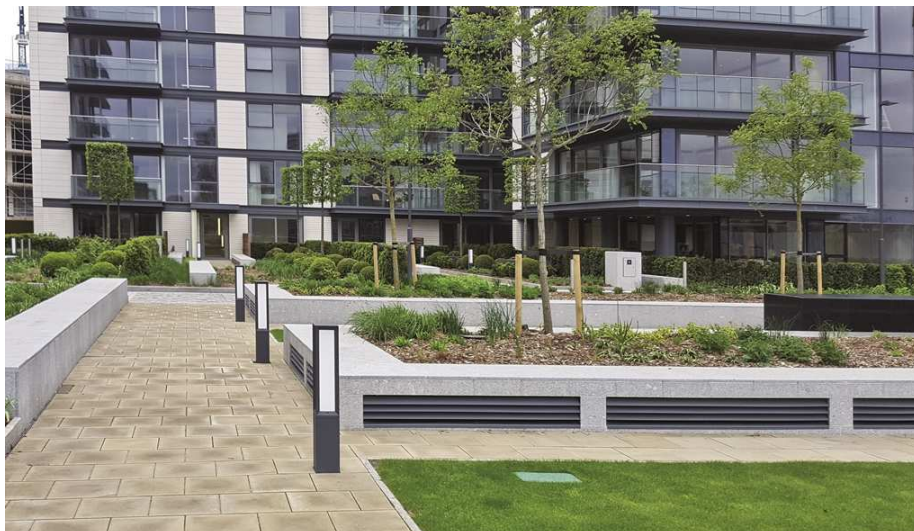
The new development with landscaped gardens was built on top of the underground car park.
