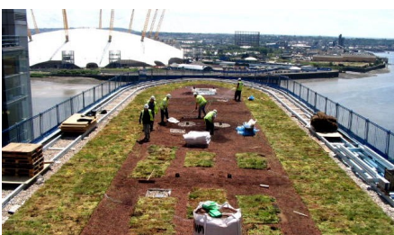
During application of the pre-cultivated vegetation mats.
