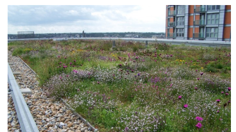
After one year the inner part of the vegetation has formed a closed carpet.
