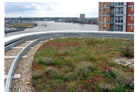
The location directly by the River Thames provides high wind load.
