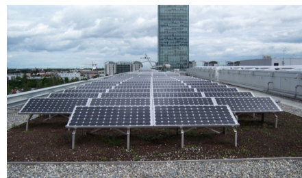
The solar panels were mounted almost to the roof edge in order to maximise the available roof area.
