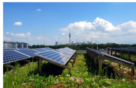
Because a green roof has a significantly lower surface temperature than a blank or gravelled roof, the photovoltaic module remains cooler over a green roof and thus a high power outcome is maintained.
