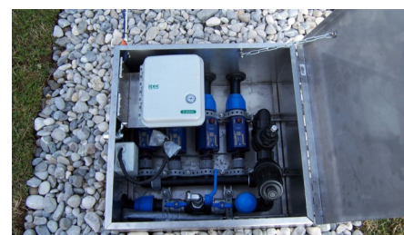
The water supply is regulated by the Irrigation Manager BM 4 meeting the demands of the vegetation.
