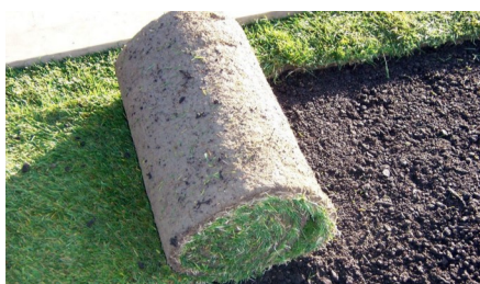
Pre-cultivated turf was laid on top of the substrate for quick covering.
