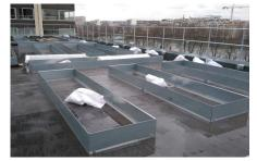
The metal frames with ca. 350 mm of height were positioned directly on the Protection Mat ISM 50, which covers the entire roof area.
