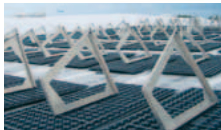
3. The Solar Base Frames SGR are placed and adjusted on the ZinCo Solar Bases.
