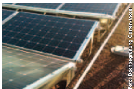
Mounting system east-west, type "Butterfly".
