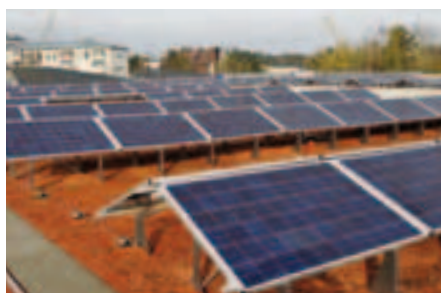
Mounting system east-west, type "Saddle".
