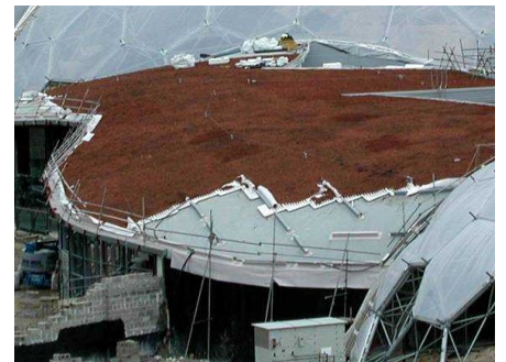
The installation of Floraset® FS 100 on pitched roofs prevents the substrate from sliding due to its profiled design. Rolled sod was used for quick covering.
