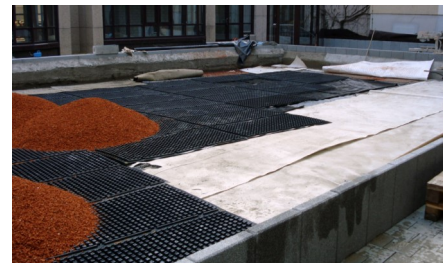
Installation of the Stabilodrain® SD 30 elements in an inner courtyard.
