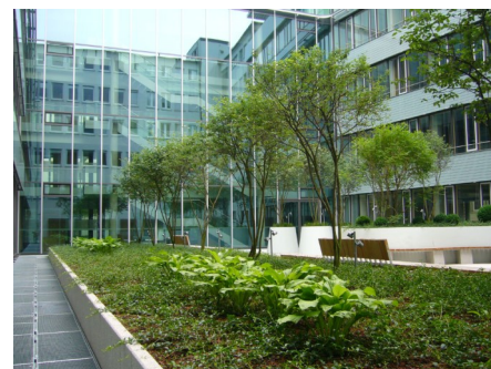
One of the green roof area of the inner courtyard short after installation...
