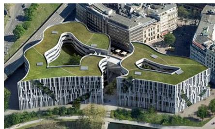
On the approximately 4.000 m<sup>2</sup> large roof surface the Floraset® FS 50 drainage element was installed. These elements are particularly suitable for large roof areas with little inclination and long drainage distances.
