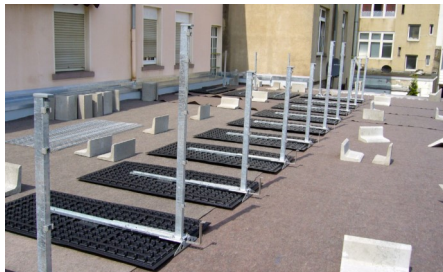
Measuring and installation of the Guardrail Base GB, as well ...
