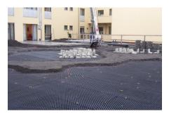
To protect the drainage elements from UV-radiation it is to be covered immediately after installation. Furthermore a protection against wind up-lift is necessary. If the further build-up is not to be applied right afterwards the elements can be weighed down temporarily by filling them with water.
