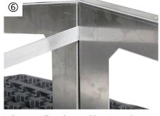
When installing the wind bracings, their exact positions according to the installation plan must be observed. The mounting is carried out like the above-described connection of the solar base frames. Only the two aluminium flat bars (pre-perforated) are to be positioned between the two frames. In addition, the two aluminium flat bars are bolted with a further M8 x 20 screw and a hexagonal nut to each other at their centre (cross-shaped).
