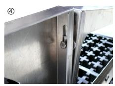
The two East-West Solar Base Frames which are arranged towards each other are to be back-mounted to each other using two screws M8 x 20, two M8 hexagonal nuts and 4 washers 8.4/30 mm (1 at each side), 1 x at the highest, 1 at the lowest point of the frame). Please consider also point 6 of these installation instructions at this step.
