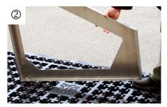
Place the Solar Base Frame SGR over the fixing points.
