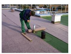
must be reported and repaired immediately. A circular piece of the protection mat needs to be cut out around roof outlets,
