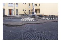
To protect the FD 25-E from UVradiation it is to be covered immediately after installation. Furthermore a protection against wind up-lift is necessary. If the further build-up is not to be applied right afterwards the elements can be weighed down temporarily by filling them with water.
