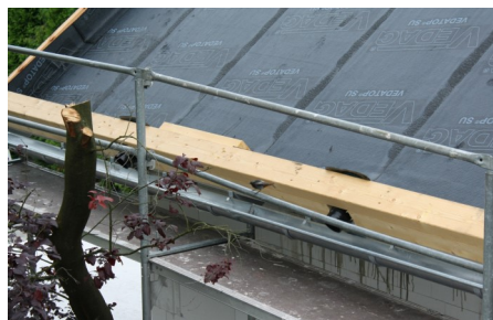
Wooden eaves up-stand prior to waterproofing.
