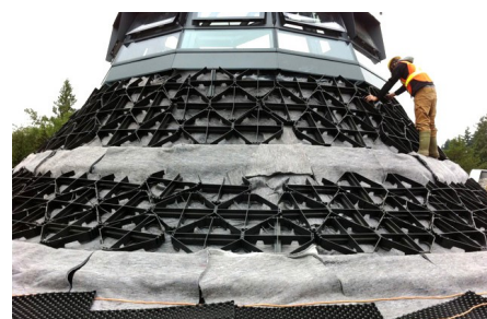
Application of the Protection Mat WSM 150.
