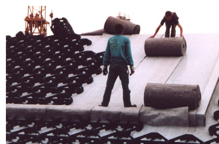
Application of the Protection Mat WSM 150.
