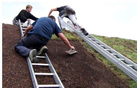
Before the vegetation mats are rolled out the substrate is to be compacted and levelled.
