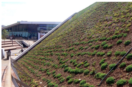
In order to achieve a dense vegetation layer, it is essential to apply two plants within each chamber of the Georaster®-elements.
