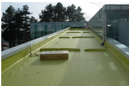
Waterproofed, interrupted shear barriers.
