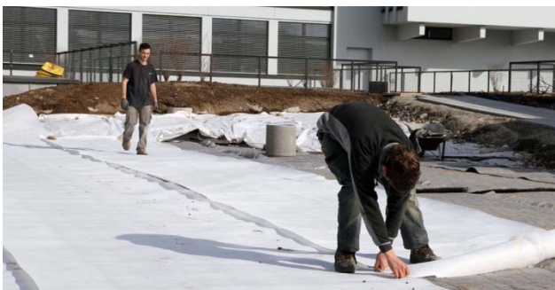
Fig. 13: Installation of the Filter Sheet PV
