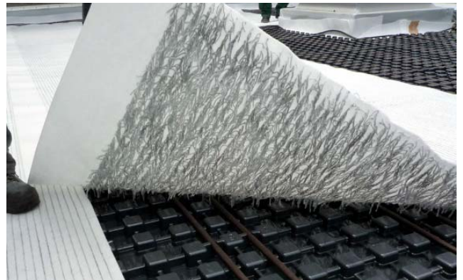
Fig. 39: Wicking Mat DV 40 installed with its wicks facing downwards
