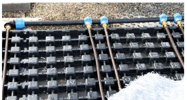
Fig. 31: Exemplary installation at the side of the supply pipe
