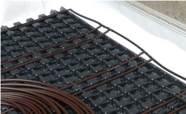
Fig. 32: Exemplary installation at the side of the flush pipe
