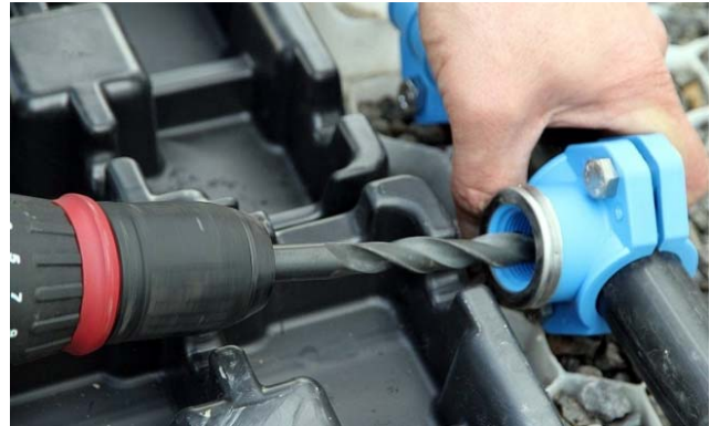
Fig. 29: Drilling the supply line
