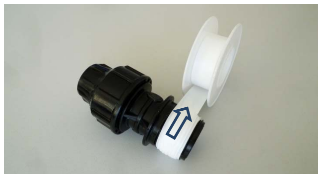
Fig. 30: Wrapping the starting piece in teflon tape
