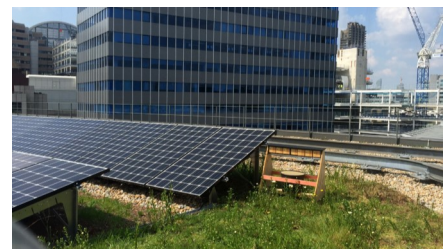
During refurbishment the old sedum roof was adapted to take a greater variety of vegetation.
