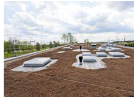
Installed system substrate "Rockery Type Plants".
