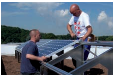
5. The solar panels are installed.
