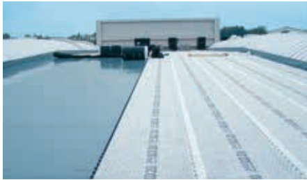
1. The roof membrane is covered with the protection, drainage and water retention element Fixodrain® XD 20.
