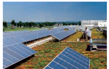
6. Roof with fully-installed solar energy system.
