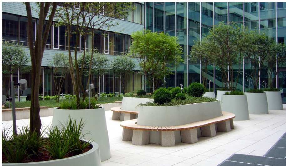
The green courtyard with planters made of glass fiber reinforced plastic.
