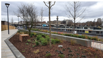
Hard and soft landscaping was installed on the podium deck in front of the Power Station using a FD 60 neo build-up. This has created vast recreational areas merging into 6 acres of riverfront park along a stretch of the river Thames which has not yet been accessible to the public.
