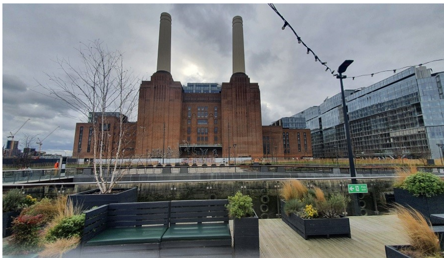
From the Thames Embankment, there is a wonderful view of the renovated façade of Battersea Power Station.
