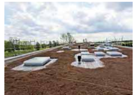
Installed system substrate "Rockery Type Plants".
