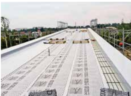
The basis is provided by the system build-up "Rockery Type Plants", in this case the drainage element Fixodrain® XD 20.
