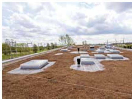
The pre-loaded system substrate "Rockery Type Plants".
