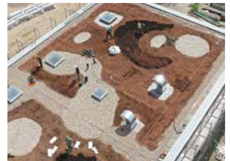
Sand, clay and gravel areas and substrate mounds provide structure on the surface.
