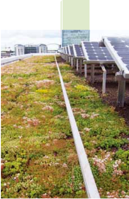
The classic area where a Fallnet rail system is used: peripheral areas, where work is required repeatedly. Once you've clicked into the runner, the work can be carried out in absolute safety.
