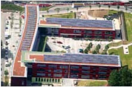
Solar energy systems are often installed right out to the roof edge to fully utilise the roof areas.
