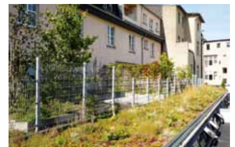
Once the Fallnet® SB 200 Rail has been mounted as a final step, there is nothing to stop the start of safe work around the peripheral areas of the roof.
