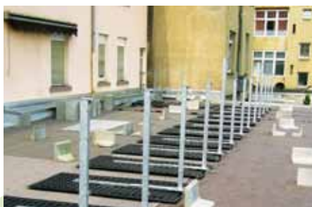
Once the protective layer has been installed onto the roof waterproof membrane, the Guardrail Base GB/GB corner are set up and the posts and, if necessary, the supports for the fixing rail are mounted.
