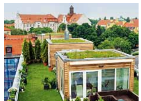
Perfectly implemented technology allows for lots of variety with an intensive green roof.
