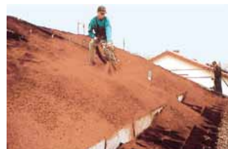
The system substrate “Heather with Lavender-light” is, e.g. delivered in a silo tanker. It is then blown onto the roof using a hose until the Georaster® elements are filled and covered up to about 10 mm over their upper edge.
