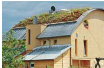
Sometimes it is a matter of structural design, as can be seen here (extreme pitch in the lower roof area), that leads to two different "coverings" being used on the same building.
