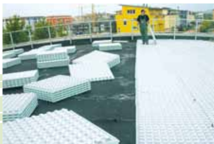
Once the Floratherm® elements were installed approx. 0,15 m of intensive substrate was blown onto the area.
