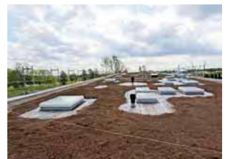
Installed system substrate "Rockery Type Plants".
