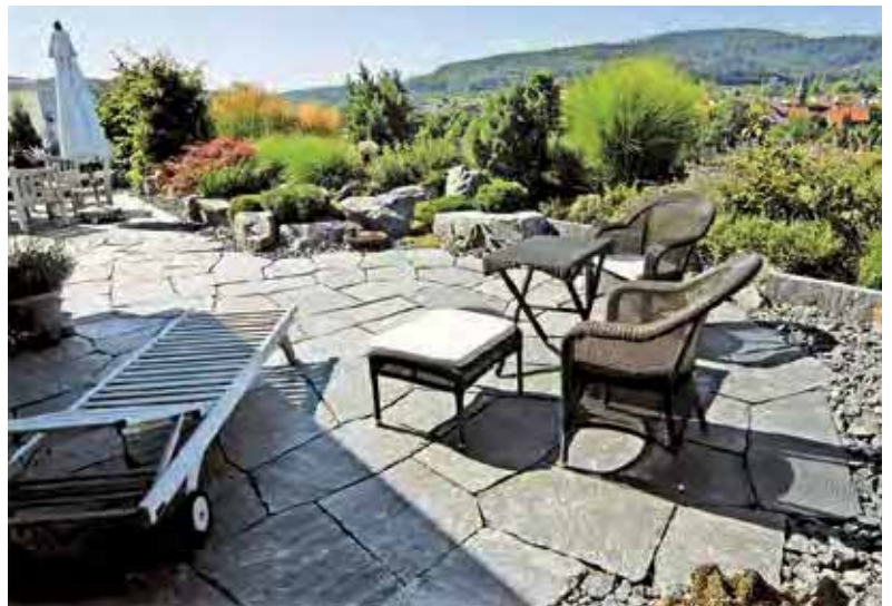
Intensive Green Roof
